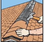
4. Center shingle cap on vent and nail. Nail line for cap shingles is to be 2"-21/2" up from edge. Continue nailing until all vent is covered with ridge caps. Be careful not to overdrive nail. Nail head should be flush with top of shingle, without indenting it. Pre-forming caps in cold weather helps avoid cracking.
