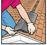
Nail one shingle cap at each end of the ridge, as with conventional application. Use End Plug in the exposed end on first and last sections of V-600, caulk in place. Center first piece on ridge and nail, keeping end of vent 1/2" from end of roof. Set 4 nails 1/2" from ends and 2" up from edge on each corner of vent, add 2 nails in center of vent 2" up from edge. Repeat this step at the other end of the ridge. For V-300, use the Folded End Cap technique (see Cor-A-Vent website).
