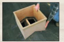
Secure the base to the roof with non-ferrous nails driven at an angle.
