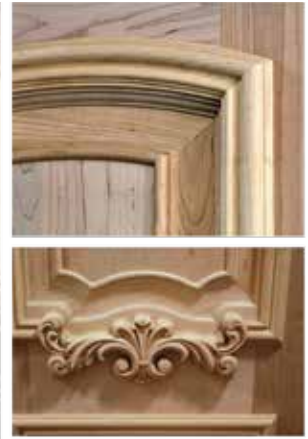
LEFT: Custom Interior Door (one of thirty units for a job) features a parquet lower panel and custom woodcarvings designed for each door. ABOVE: Two panel mouldings frame upper and lower panels creating soft but dramatic framing, which fits perfectly with the custom carving.
