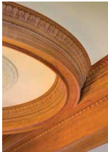
ABOVE: The ultimate architectural element – curved beams merging with straight beams. The straight handcarved mouldings are manufactured from Cherry and curved carved mouldings manufactured from resin – and who can tell the difference? Resplendence. Grand.
