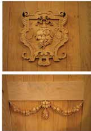
LEFT: Fanciful pantry door built by our Custom Shop features rail and stile frame with vertical panels. The deeply carved custom woodcarvings are based on the clients' photos.
