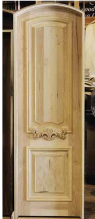
LEFT: Custom Interior Door (one of thirty units for a job) features a parquet lower panel and custom woodcarvings designed for each door. ABOVE: Two panel mouldings frame upper and lower panels creating soft but dramatic framing, which fits perfectly with the custom carving.
