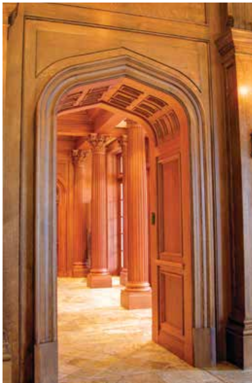
ABOVE: The ultimate architectural element – curved beams merging with straight beams. The straight handcarved mouldings are manufactured from Cherry and curved carved mouldings manufactured from resin – and who can tell the difference? Resplendence. Grand.
