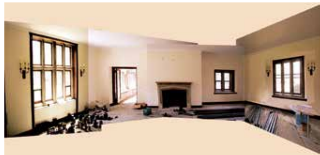
Design Services requested with these jobsite conditions
