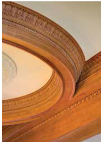
ABOVE: The ultimate architectural element – curved beams merging with straight beams. The straight handcarved mouldings are manufactured from Cherry and curved carved mouldings manufactured from resin – and who can tell the difference? Resplendence. Grand.
